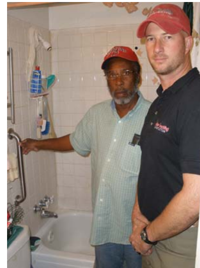
Mr. Wraggs shows the grab bar installed by Matt Strecker Strecker Remodeling
